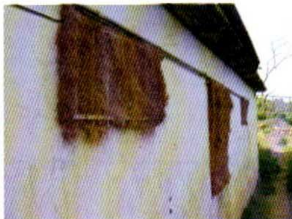
Fig. 1b. Mud house with evaporative cooling pad system
